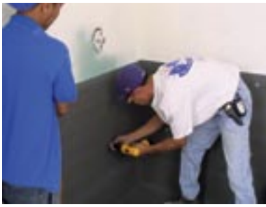
wedi building panel is applied to the wall over gypsum or directly to stud.
