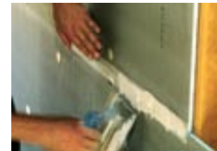
In dry areas, the seams can be treated with an alkali resistant fiberglass mesh tape by wedi.
