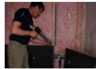
A continuous 1/2" bead of wedi joint sealant is applied on the foam edges of a wedi building panel before another panel is joined butted tightly.
