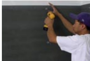
Fasten wedi building panel into place with wedi screws or nails with washer-heads.
