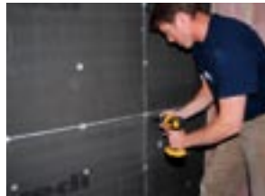
Apply wedi fasteners at a rate of 1 per every 12 inches with an extra fastener right in the seam to provide a flush transition. On a ceiling, the fasteners are set at a rate of 1 per every 6 inches. The washer heads are dimpled below the surface of the wedi building panel.
