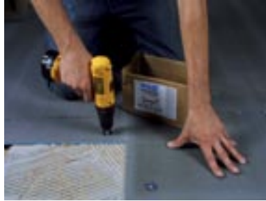
Fasten with wedi fasteners.
