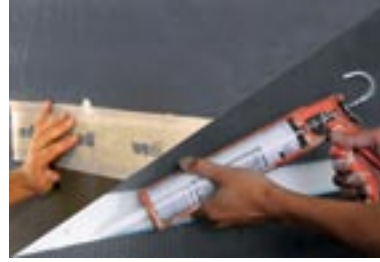
wedi polyurethane sealant or wedi waterproof tape is applied on the seams and fastener points.
