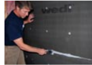
All excess wedi sealant is spread flat over all joints using a putty knife. Where needed, an extra bead of sealant is applied on top of the joints and spread flat. The joints should be covered a full 3/4" on both sides of the seam.
