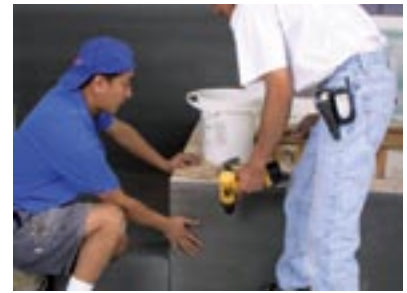
On solid backing constructions use a modified mortar and wedi fasteners to apply wedi building panel.
