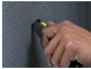
Using only a utility knife wedi building panel is effortlessly cut and shaped.
