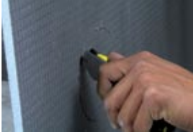
Using only a utility knife preparing the shower is a snap.
